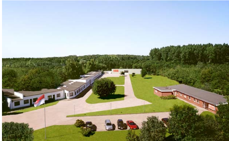
5 - The Clear & Clean plant for cleanroom technology, located on a 3,2 acre site in Lübeck
